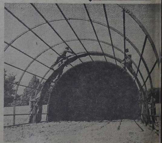
PORTABLE SHELTER —This medium-sized portable shelter, of aluminum and covered with fabric, may someday replace tents and house both troops and equipment. The shelter is being tested here and is being evaluated by Landing Force Development Center. (Photo by Cpl. J. L. Hyppa)
