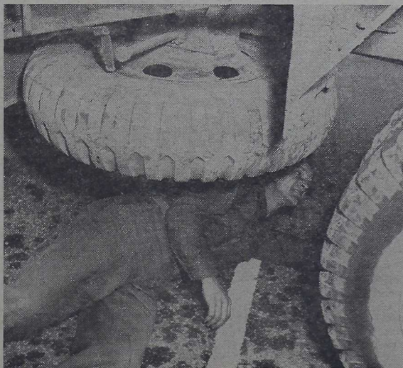
BIG WHEEL —SSgt. W. P. Mihalovich, "B" Co., 2d MT Bn., 2d Marine Division, checks the torsion bars and drive shaft of one of the many vehicles stopped for inspection by the joint roadmaster inspection team which set up operations in the parking lot opposite Goettge Memorial Field House last Monday. (Photo by LCpl. J. Varga.)
