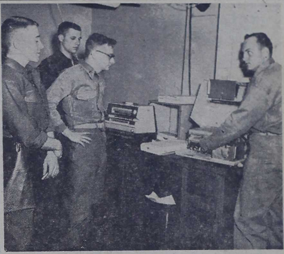
OPERATIONAL PROCEDURE —Cpl. Larry Elmen, right, instructs Pfc's Omer Windham, Philip Cangelosi and Michael Shea, left to right, in the operation of a photostatic reproduction machine. The machine turns out photostatic copies of small documents in less than four seconds. (Photo by Pvt. C. D. Vardaman)
