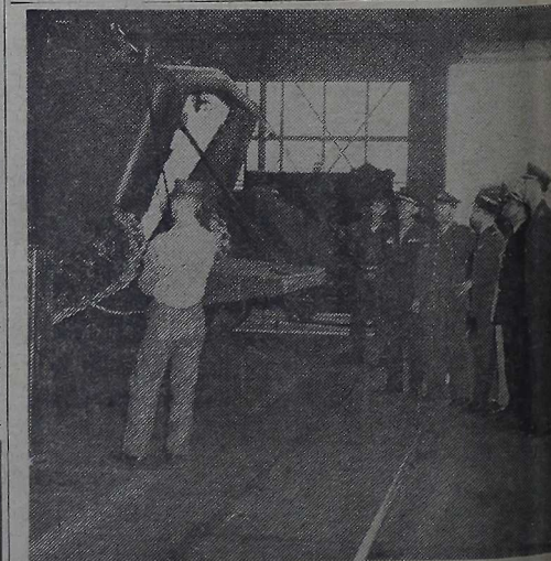
UP SHE GOES—Six visiting Allied officers who arrived here last week for a two-day tour of the base facilities look on as an overhead-bridge crane lifts an LVT-P5 amphibious tractor into position for operational maintenance. Two Marine foreground guide the 34-ton vehicle into place. The officers represent Allied nations in South America, Europe and Asia. (Photo by Pfc C. B. Vardaman)
