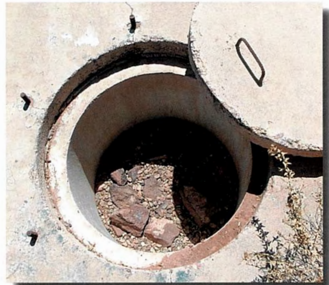
One of the manholes at a location marker.
