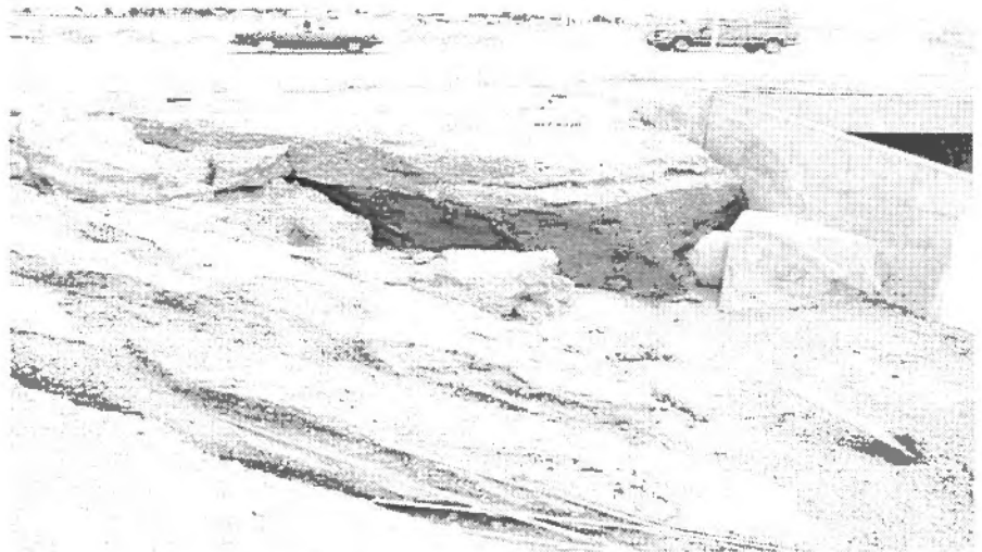
Looking upstream at an area under construction. This is a transition area where the channel is changing from open rectangular to trapezoidal.
