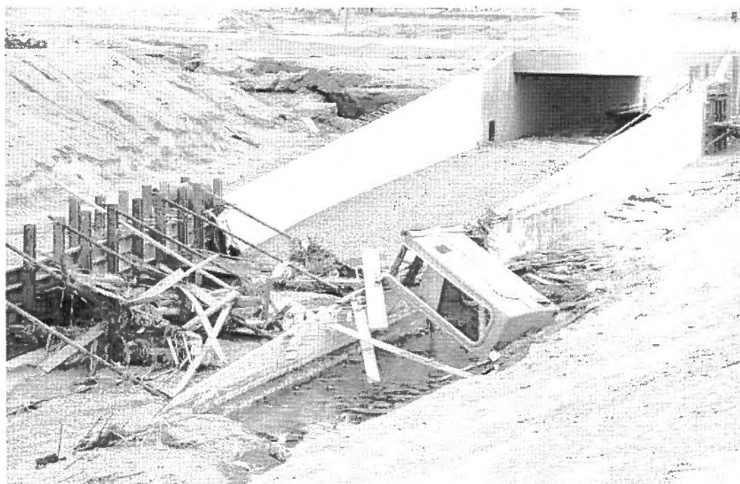
The south side of the channel, downstream of the Decatur crossing which captures some of the scour damage which was typical in many areas of the City, this just happens to be at our channel.
