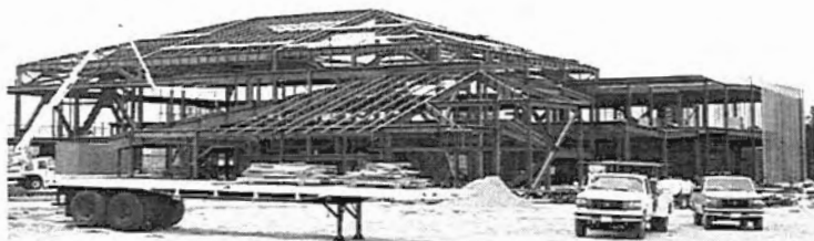
The control center's steel skeleton is ready for its frame to be fleshed out.
