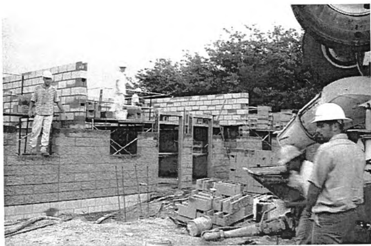
The concrete flows and workmen erect masonry-unit walls as Nellis AFB's newest dormitory sprouts in the upper Mojave Desert of Southern Nevada.
