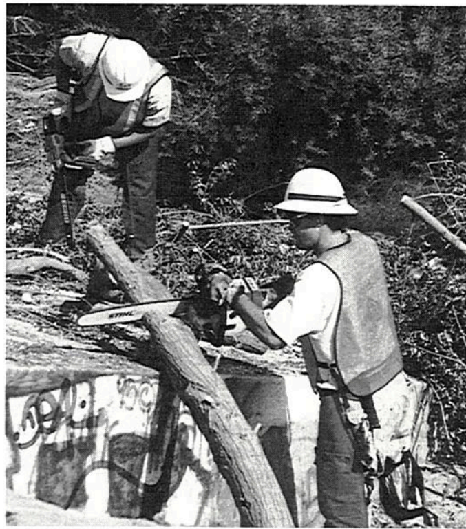
Sometimes it takes two people to get the job done.
