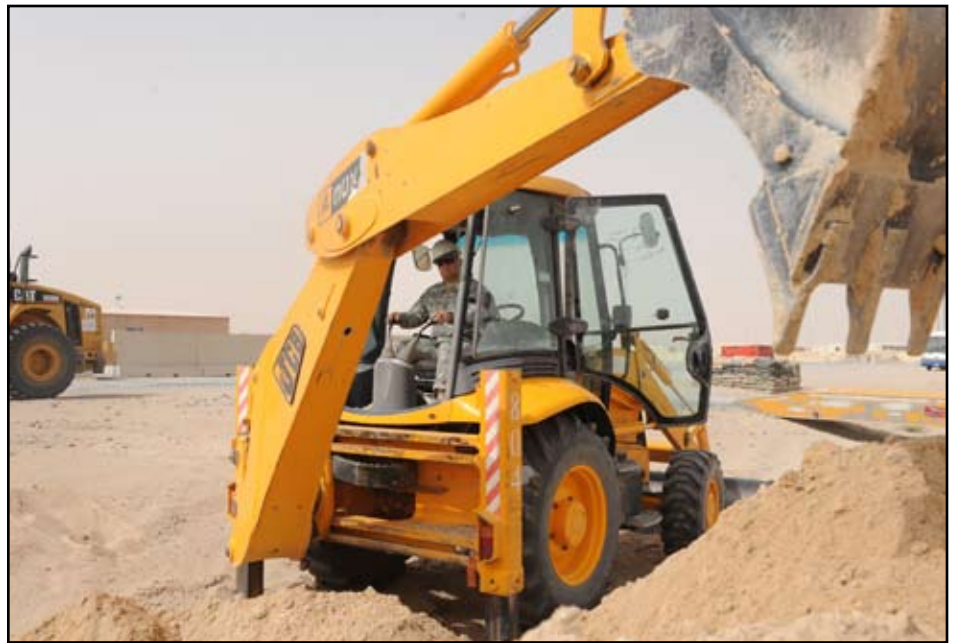
Sgt. Keith Reedy improves the roads at the Life Support Area, Kuwait by cleaning out the drainage ditches with a backhoe. (photo courtesy of U.S. Navy)
