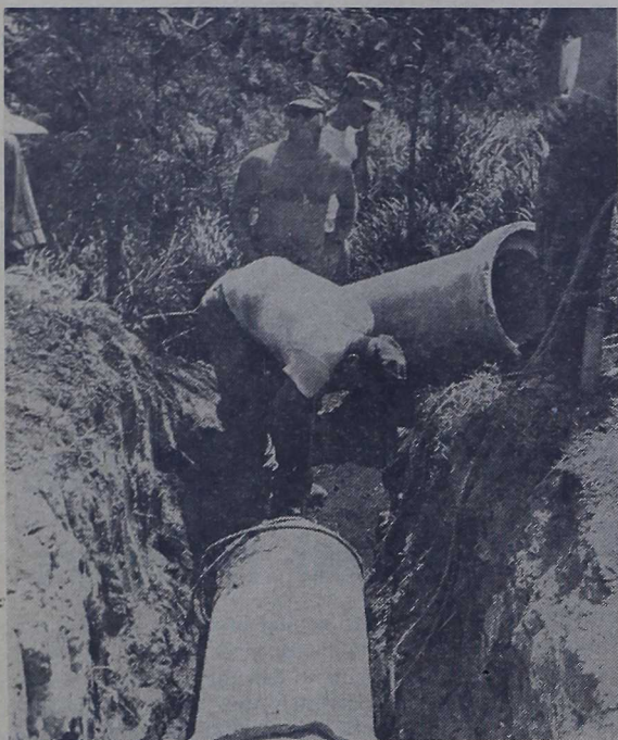
UNDERGROUND WORK —Cpl. Ray Hagen, foreground, clears the way for a section of underground culvert through the thick Vieques undergrowth. Hagen and other reservists trained with the 8th Engineer Bn. for two weeks on the Caribbean island. Working with Hagen on the project is LCpl. L. Ballant and Pfc Mick Maskrey, respectively.
