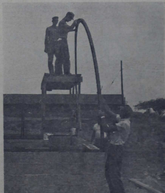
HOUSE BUILDERS —Five Orlando, Fla., reservists help in the construction of a quonset hut by guiding a steel rib into position and attaching it to the cement blocks which form its base. Holding the rib in place at the floor level are Pfc Glenn Hennig and LCpl. Charles Bowen (background). Guiding the rib into position at the roof level is Sgt. Jack Grover, left, and LCpl. Fred Hall. SSgt. Charles B. Keene, between Bowen and Hennig, acts as supervisor for the construction.
