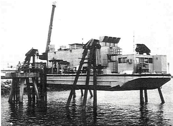
Dolphins suspend equipment-laden barge above the water to improve stability for the system's piping, stastability for system.
