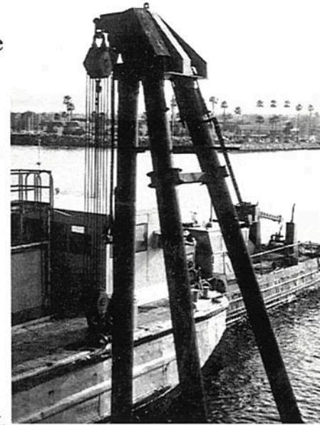
Called dolphins, these steel support assemblies are used to hoist a boat out of the water.
