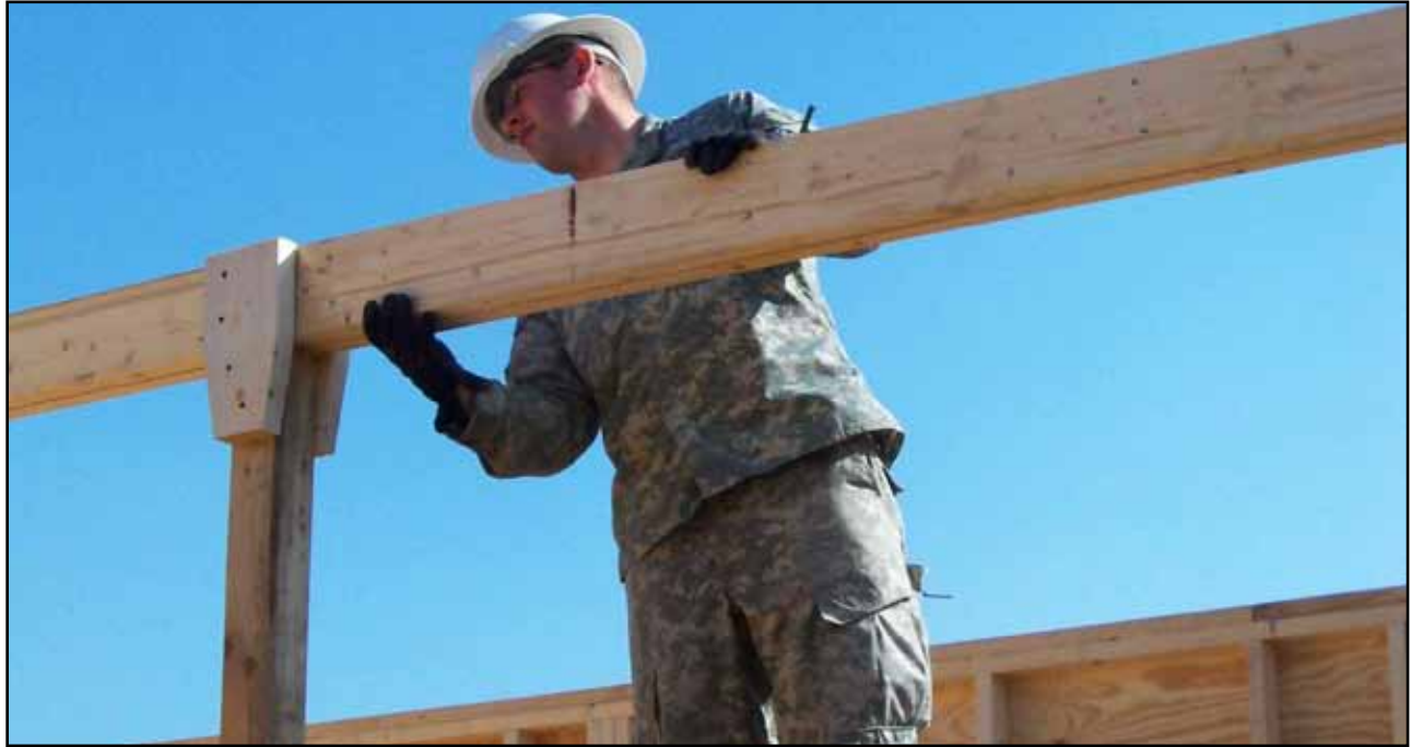
Pvt. 1st Class Jeff Rochefort from Munising, Mi., a member of 1434th Engineer Company, works to install a support beam Jan. 7 at Joint Security Station Nasir Wa Salam. The 1434th Eng. Co. is working to construct an expansion to the main gym at NWS. When complete, the expansion will be able to accommodate the additional Soldiers that are stationed there.
