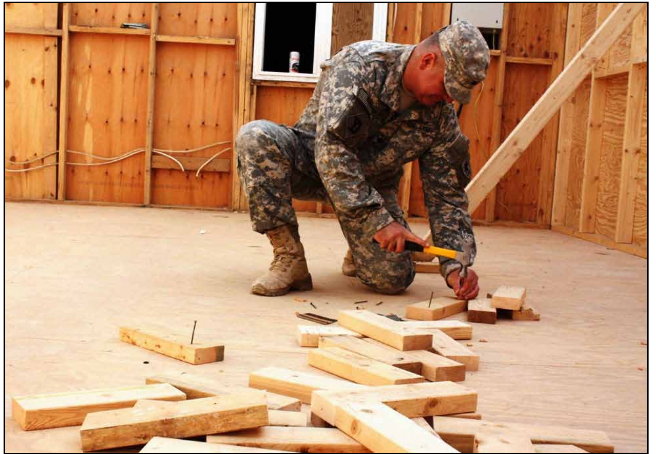
Spc. Eric Zihlman, a native of Grossepointe Park, Mich., assigned to 1434th Engineer Company, hammers nails into wood blocks that will be used to attach trusses to the roof of a new addition to a gymnasium at Camp Liberty. The addition, planned and built by Soldiers of 101st Engineer Battalion, will more than double the current size of the facility.
