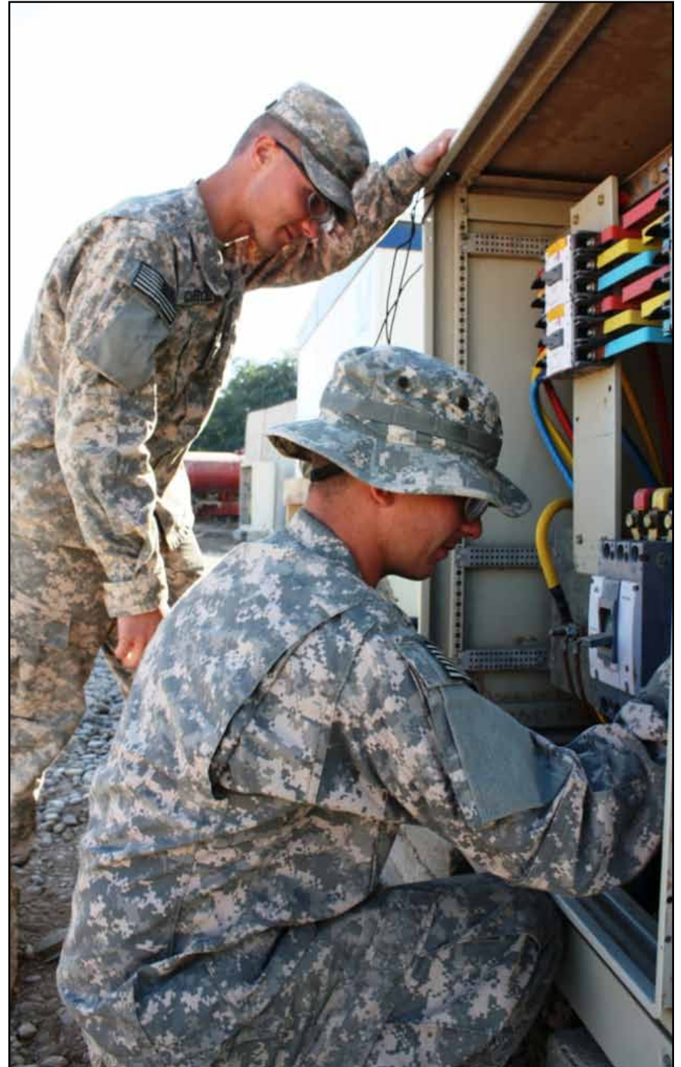
Prior to turning on the electricity, Spc. Brandon Burgess, of Hammond, Ind., with 317th Engineer Company, makes sure all connections are secure while Pfc. Sean Carroll of Dyer, Ind., 317th Eng. Co., observes the process. Soldiers from 317th Eng. Co., are providing power to new housing units for Soldiers of 10th Mountain Division at COS Carver.
