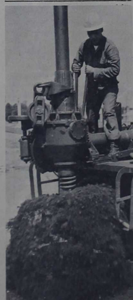
"DIGGING IN" —With LCpl. Michael Feeney at the controls of the V-18 Auger, it takes no time at all for members of Radio Relay and Construction Co., 8th Comm. Bn., to install telephone communication lines at New River Air Facility.
