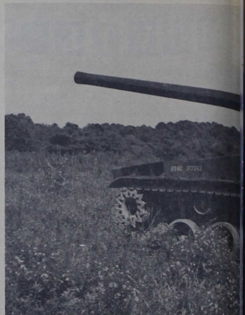
LONG AND LETHAL—Pictured above is the 155mm self-propelled gun with a range of 23,400 meters.
