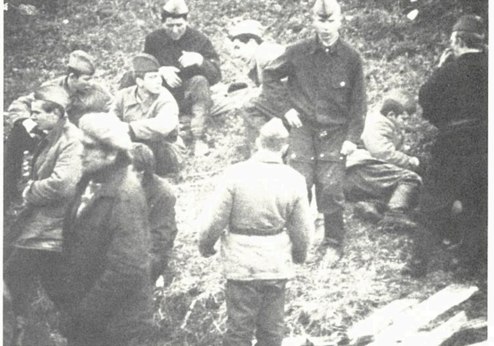
Railroad work crew at Krasnoyarsk Station. Russian soldiers are used as laborers, in this instance.
