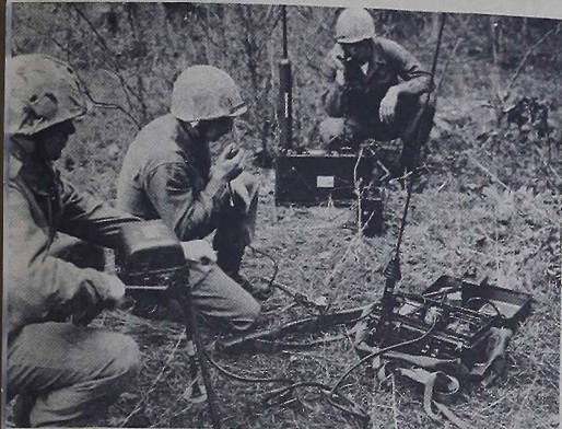
TEST SINGLE-SIDEBAND RADIO —Members of 2d Air and Naval Gunfire Liaison Co., Force Troops operate the AN-GRC-9 radio, foreground, while a radio operator, rear, tests the new AN/PRC-47, single-sideband radio which is replacing the AN-GRC-9.
