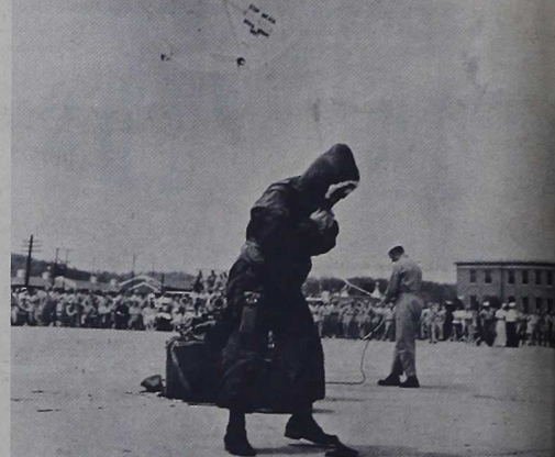
SADDLE UP —Maj. Larry P. Charon makes final adjustments to his flight suit just prior to being snatched from the ground by an S2A twin-engine naval aircraft during a demonstration of the Fulton "Sky-Hook" June 9, at the Marine Corps Air Station, Quantico. Adjusting "risers" to the Major's right is Parachute Rigger First Class Vasseur of the Naval Aerial Test Center, Patuxent River.
