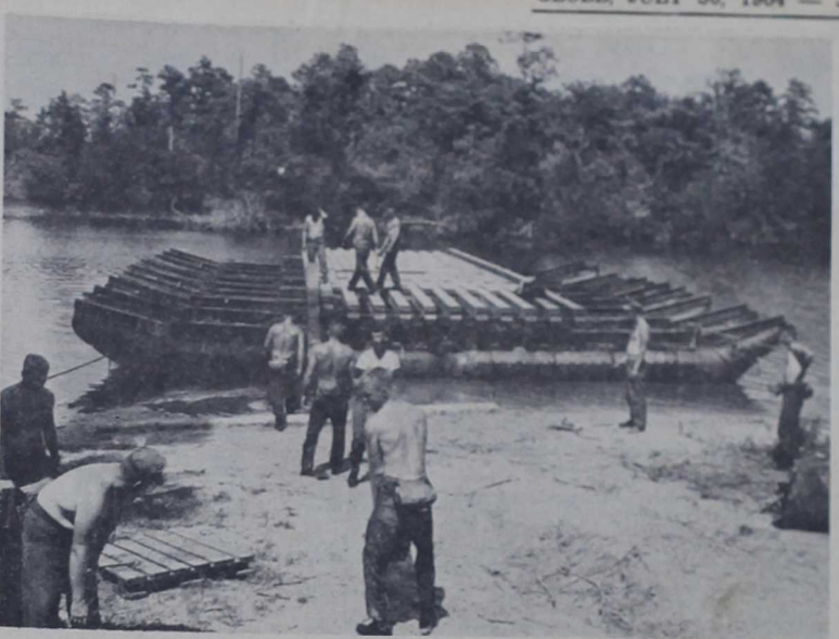
RIVER BARGE —Members of 2d Bridge Co., Force Troops, dismantle the raft they constructed to float their gear 15 miles down the South-west Creek to a bridge construction site. The pontoons will later be used to support the proposed bridge.
