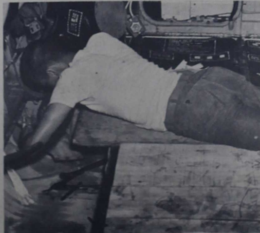
BULLET HOLES —Up come the floorboards and down go the metal patches as Cpl. Hugh D. Sisco, a Marine metal-smith, covers bullet holes in the bottom of a UH-34D.
