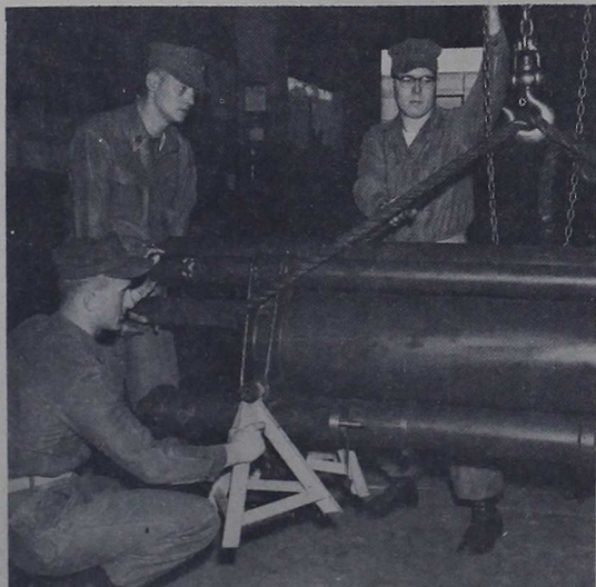
GUN POSITION—Reserve Marines of the 1st Ordnance Field Maintenance Company, Columbia, Pa., are setting in position the recoil mechanism of a 105mm Howitzer for repair. These Marines are receiving two weeks annual field training here.
