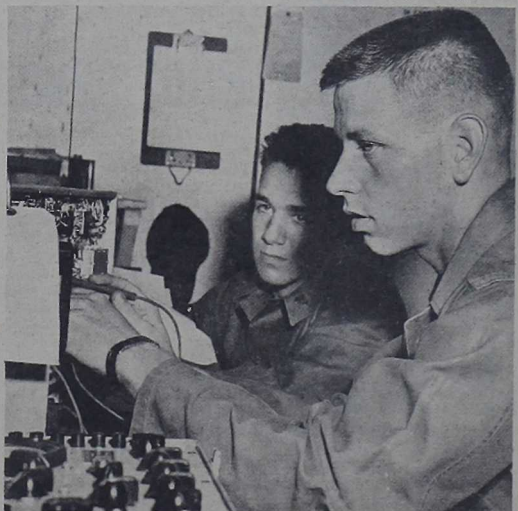
CHASING GREMLINS —Cpl. G. T. Weiss (right), probes wire and transistor maze of radio transmitter under the guidance of Cpl. V. D. Puso. By using test equipment in left foreground, discrepancies are located and repairs made. Weiss, a trained Radar Repairman, is undergoing cross-training in Radio Repair from Cpl. Puso, platoon maintenance chief.
