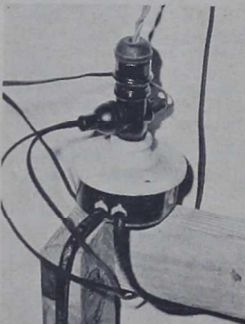
OVERLOADED CIRCUIT — Electrical fires rank as the second major cause of fires at Camp Lejeune.
