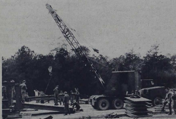
BUILDING A BRIDGE - 10th Engineer Marines use their know-how and a crane to assemble the M-6 Bridge. The bridge is strong enough to accommodate the heaviest equipment, including a tank.
