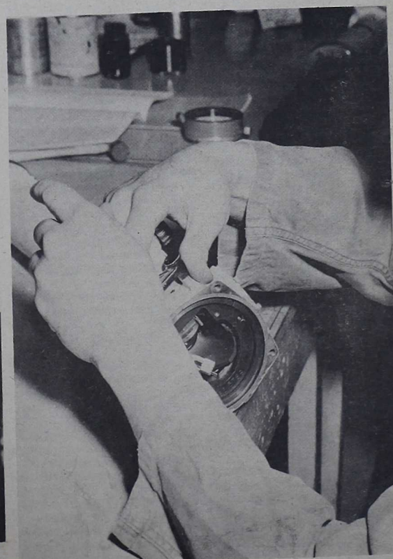
THE SKILLED and experienced hands of a specialized Marine service the sight mechanism from a Self-Propelled Howitzer.
