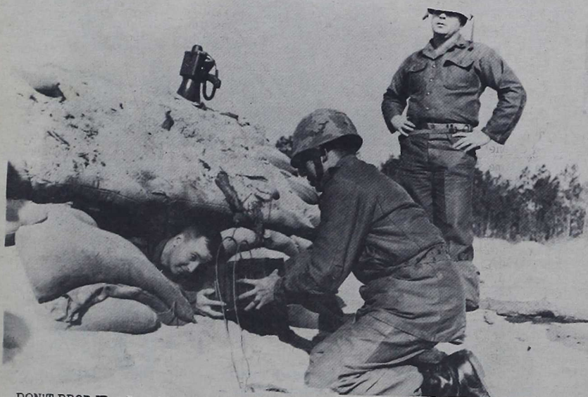
DON'T DROP IT — Demolition instructor supervises students emplacing a charge of TNT into a sandbag bunker. Short minutes later the
