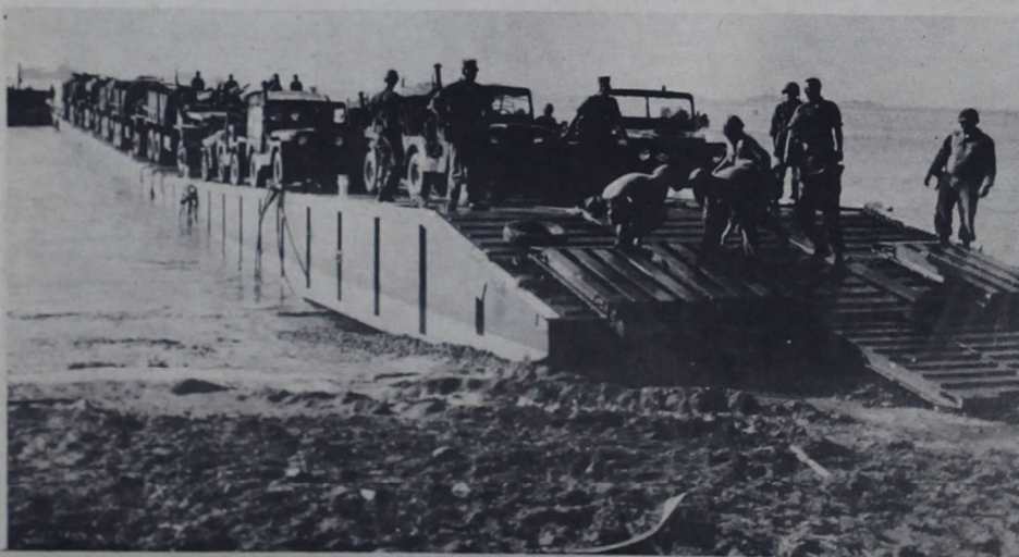
FLOATING DOCK — Men from the Causeway Platoon, Naval Beach Group, part of a Shore Party Team when Task Organized, complete the construction of a Pontoon Causeway. The Causeway is one link for supplies moving from Ship to Shore.
