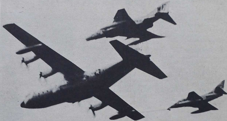
TANKING UP - An F-4 (left wing) and an A-4 nose in for demonstration of in-flight refueling behind a C-130.
