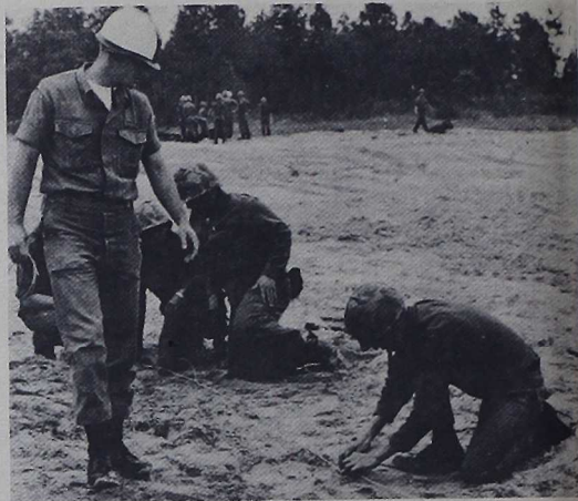
WIRING --Sergeant Sparks (standing) checks the tie-ins as Seabees connect the detonation cord for three 40 lb. ammonium nitrate cratering charges.
