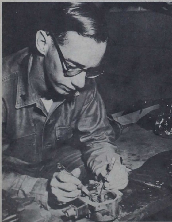
DELICATE OPERATION — Cpl. John L. Zimmer adjusts the breaker points on a distributor. The trained mechanics of the battalion are conducting constant maintenance to keep the rolling stock in top road condition.
