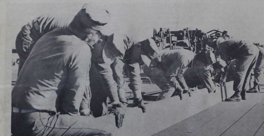
TEAMWORK — Combat Engineers of "B" Company, 8th Engineers, install a section of AM-4 aluminum matting on Bogue Field's Short Airfield for Tactical Support (SATS). The company
