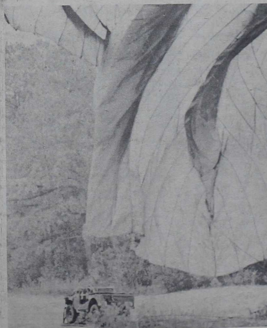
SILK SHEET -- After landing, a jeep is almost engulfed by its parachute. The huge silk sheet weighs 250 pounds and the canopy is 100 feet in diameter.
