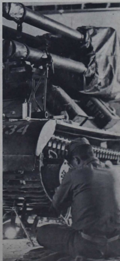
KEEP THEM ROLLING - The same men who operate the tank-killing Ontos must also make sure that its weapons and running gear are kept in first class condition.
