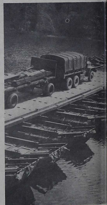
TRUCKS AND TRAILERS haul bridge materials, including 44-foot long pontoons. This is one of the training sites at Camp Lejeune.
