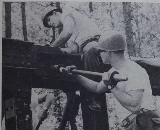
RESERVE MARINES line up a truss panel to pin it in place on one of the several types of bridges they learned to assemble at Camp Geiger.
