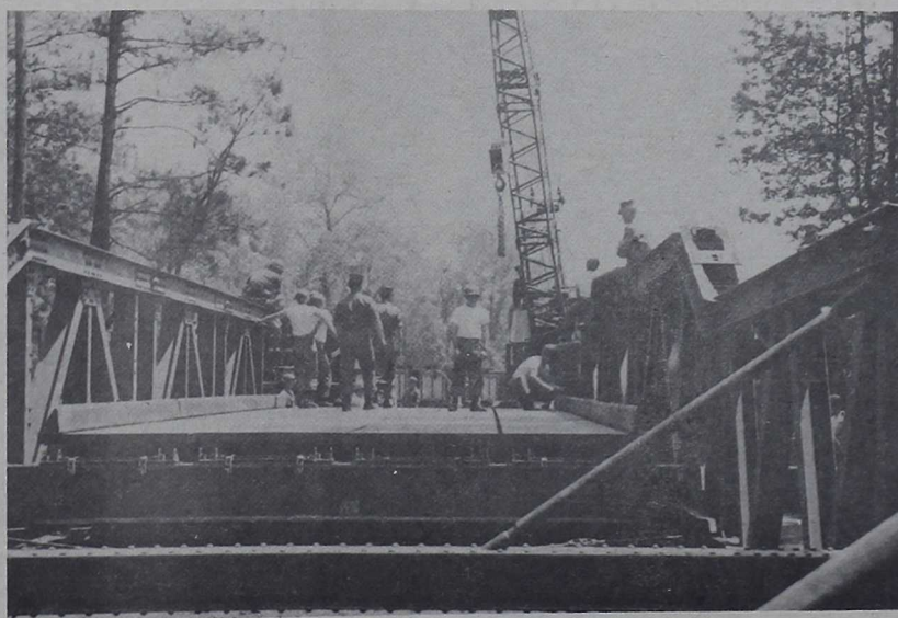
RESERVE MARINES lay the aluminum flooring in a fixed highway bridge.
