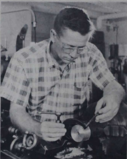
MACHINIST, Mr. O.W. Gillette, checks the tolerance of a turned shaft.
