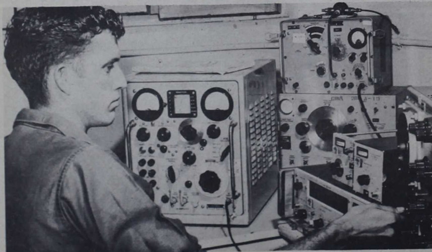
A MAZE OF dials are all part of the daily routine for SSgt. Donald Kennedy while conducting electronic equipment checks. Here he tests a signal generator. With this and other electronic calibration apparatus the lab tests equipment from all major East Coast Marine Corps units.
