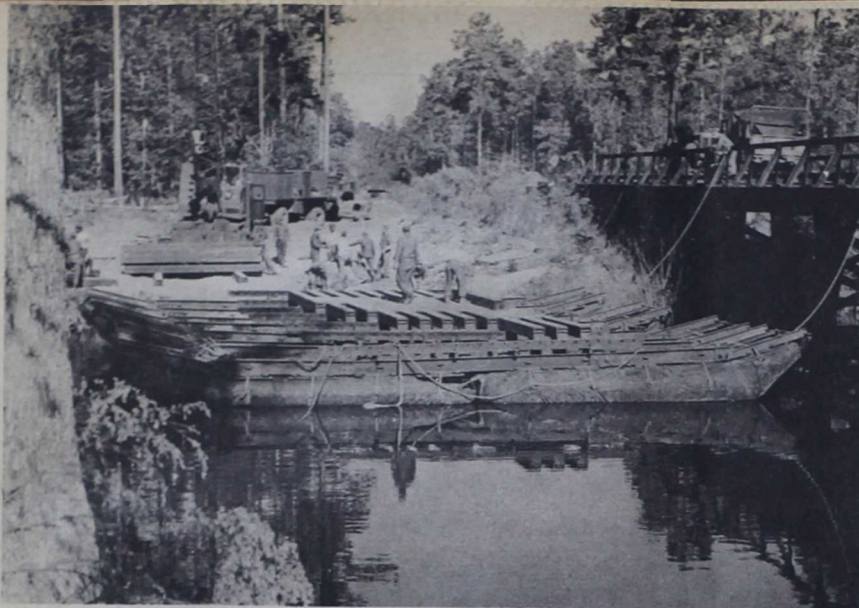
BRIDGE BUILDERS from the 2d Bridge Company place light strans of cover over pontoon floats during field exercises.
