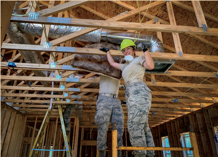
U.S. Air Force Airman Destiny Carl, 177th Civil Engineering Squadron, installs insulation wrap on a heating, ventilation, and air conditioning duct at Camp Kamassa in Crystal Springs, Miss., Aug. 1, 2019. (U.S. Air National Guard photo by Capt. Nathan Gorey)
