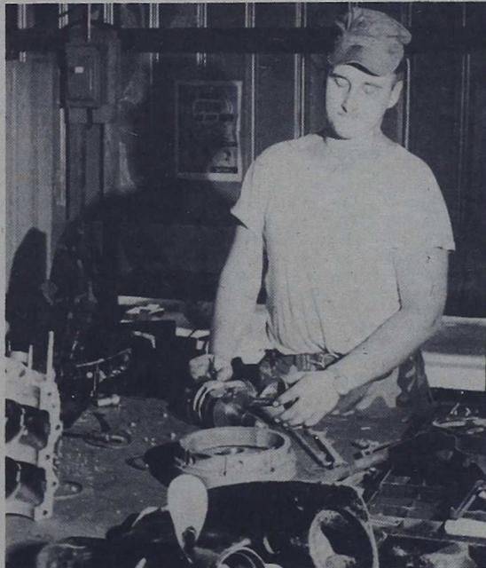
**ENGINE REPAIR** — Besides providing third and fourth echelon maintenance for generators, the Engineer Maintenance Company Generator Shop fixes all small engines, including the outboard motor that Corporal Carl Kuchenbecker is repairing.
