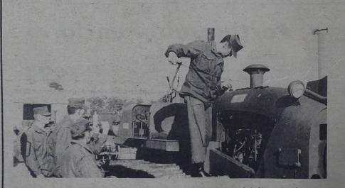
OH, CHECK — An I.G. inspector checks the level of oil in a bulldozer during a technical inspection of 8th Engineer Battalion, Force Troops-2d FSSG.
