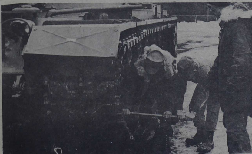
TANK TRACK — Tankers of "A" Co., 2d Tank Bn., attached to 1st Bn. (Rein), 8th Marines, at Fort Drum, N.Y., tighten a track center guide on an M48-A3 Tank during exercise Alpine Warrior, Feb. 27 to Mar. 1.
