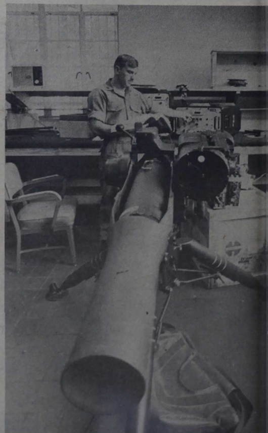
TOW TESTER — Cpl. John Hicks, a TOW technician with (TOW) Co. prepares to calibrate the missile guidance system antitank TOW.
