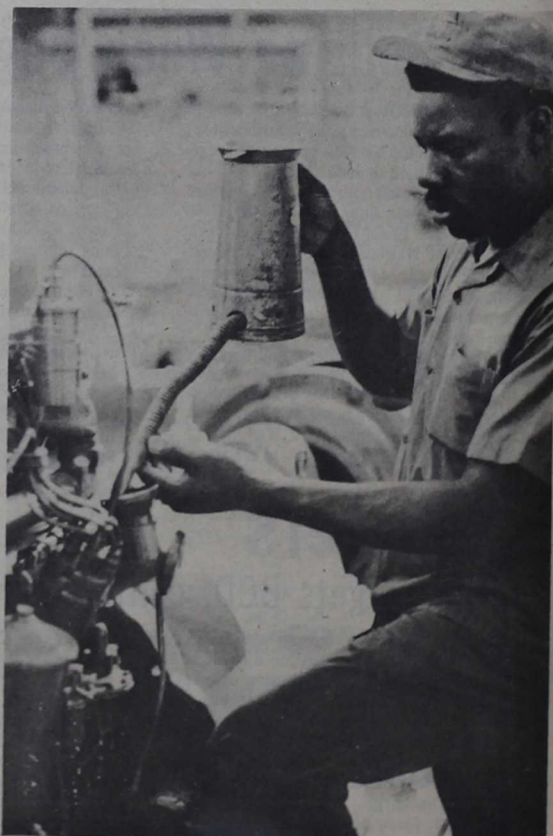
JUST IN CASE — Auxiliary gasoline engines receive weekly checks by water plant employees at Camp Lejeune, N.C., George D. Milton oils one of the engines used to supply emergency power to water pumps. (USMC photo by SSgt. Arvel "J" Edward Hall)
