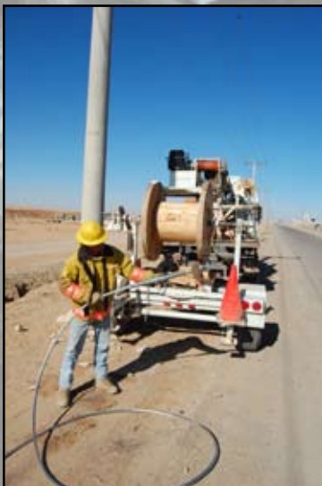
Contractor Michael Gallagher splices a grounding conductor on a feeder line along Perimeter Road at Contingency Operating Base Q-West, Iraq, Jan. 23. The line will improve electrical safety around the base. Electrical fires are one of the most common preventable accidents in theater bases.
