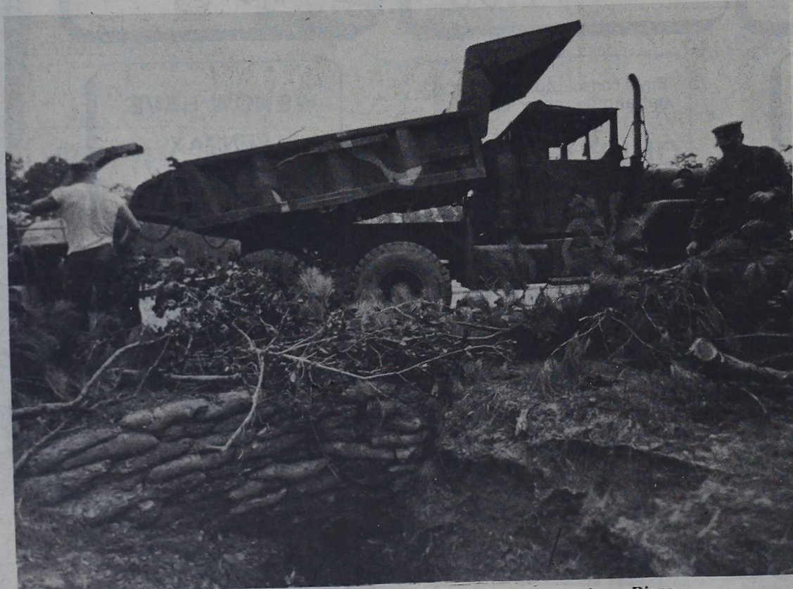
Dump truck drivers remained busy moving all of the debris piled up by Hurricane Diana.
