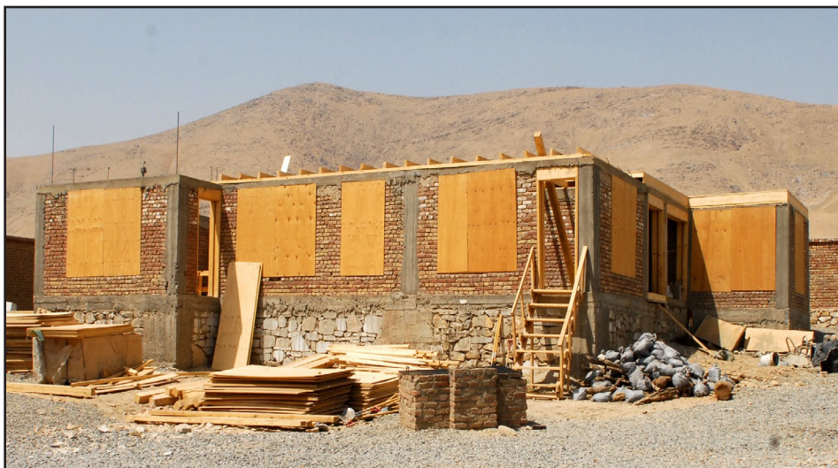
The New Command Post is near completion at COP Blackhawk. The brickwork was the only portion of the structure completed when the Soldiers arrived in April. Since that time, Soldiers have worked countless hours on construction and laying concrete to level the facility and replace the rock pit that once stood as the flooring of the building. (Photo by Sgt. Rob Frazier).
