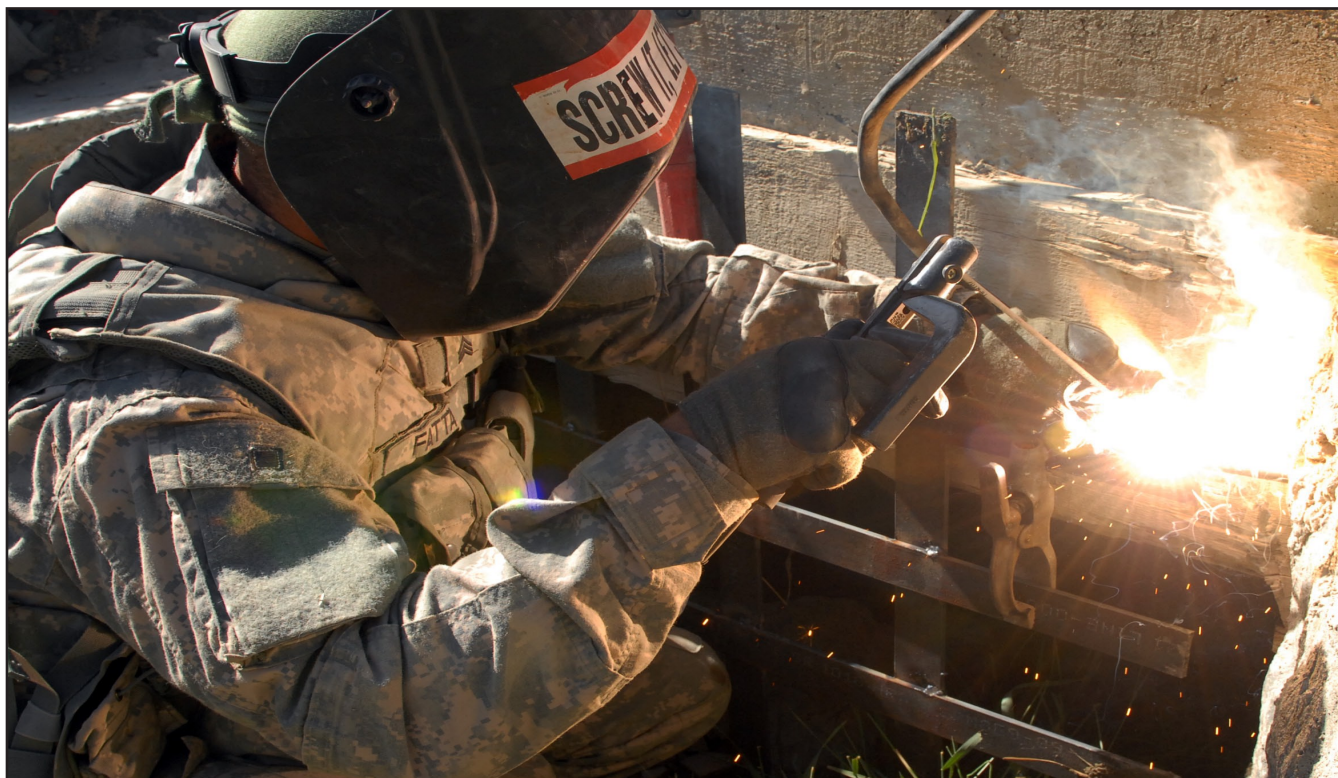
Sgt. Salvatore Fatta, a welder with Company G, 4 th Battalion, 25 th Field Artillery Regiment, welds a steel grate over a culvert in Wardak province, Oct. 23. "I think this is my part of the fight," said the Buffalo, N.Y. native. (photo by Spc. Matthew Thompson).
