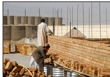
Local nationals apply mortar to the bricks of a new building at Forward Operating Base Altimur. Soon, these workers will be able to implement the same skills in their own villages with the creation of Extreme Make Over in Logar province, Afghanistan.
