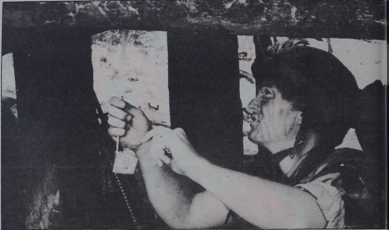
Private First Class Curtis G. Goad, Charlie Company, 2d Combat Engineers, 2d Marine Division, calculates the amount of explosives necessary to blow the bridge. (Photo by LCpl. V. S. Bode)
