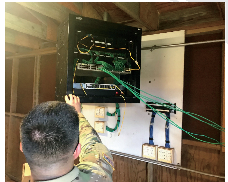
During the exercise, Soldiers configured network switches, ran fiber and Ethernet cables to all locations, and while troubleshooting information systems.
