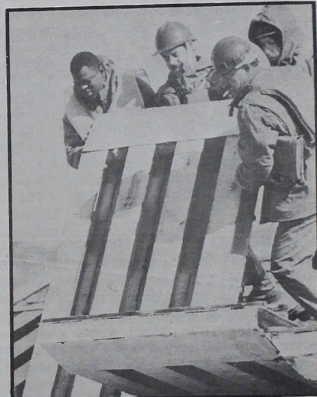
WORKING TOGETHER — Marines and Sailors work together to set the pieces of causeway ramp so vehicles can drive to shore.
