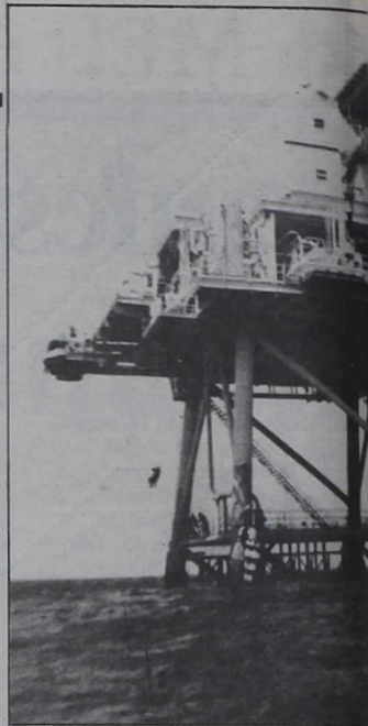
The top of the 24th MEU oil platform. Above, A paratrooper is seen in the landing quarters.
