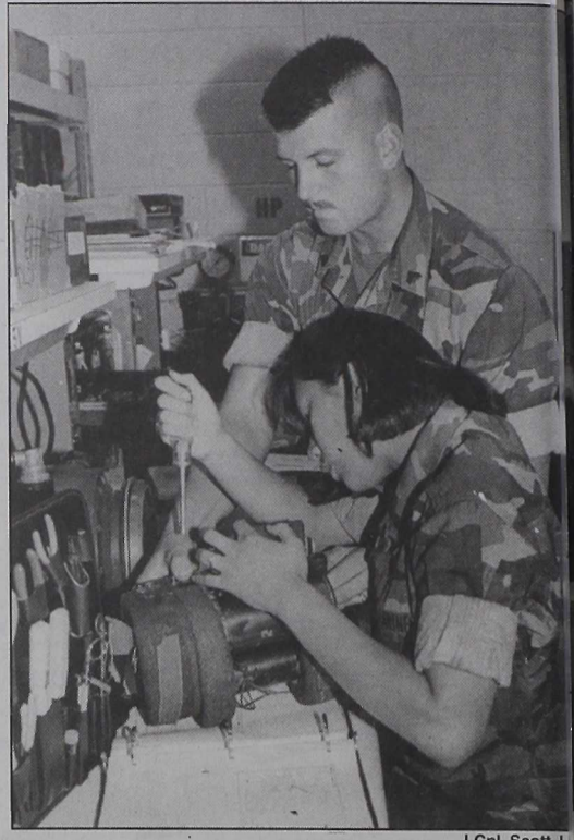
LCpl. Stella Y. Sabourin, missile technician, OMC, works on sight of a Dragon missile as Cpl. Joseph Stephenson steadies.
