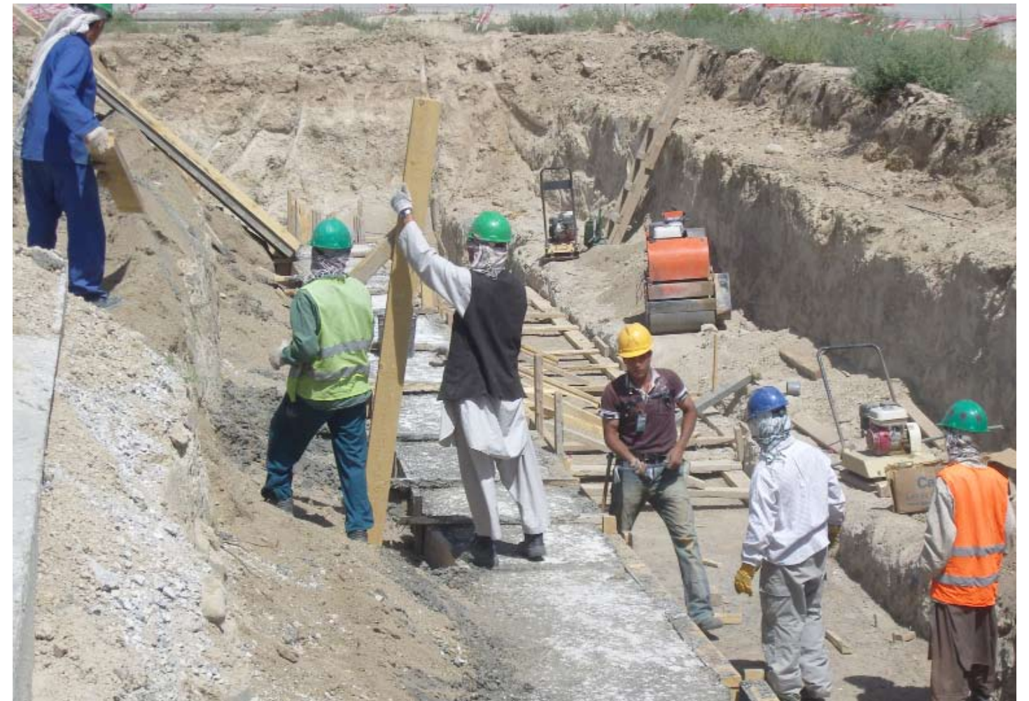
Workers make sure to build drainage for the new road. The drainage will allow water to drain more readily and cause less flooding.
