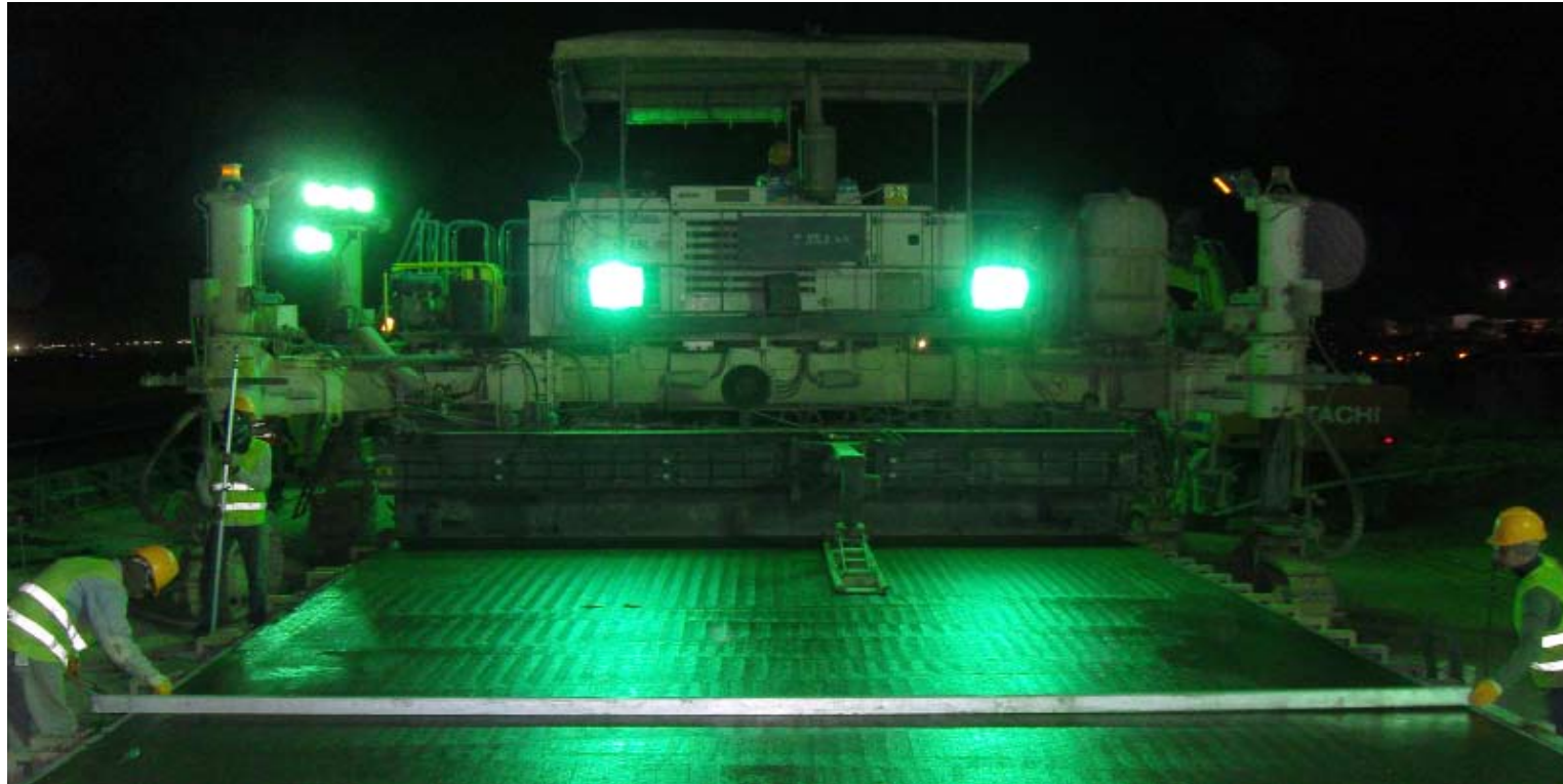
A paving machine places a fresh concrete lane while workers ensure it is level.
