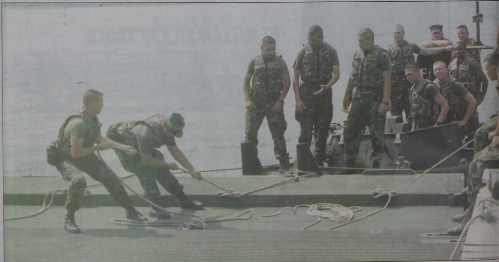
Marines secure sections of ribbon bridge to provide safe crossing for foot and vehicle traffic.
