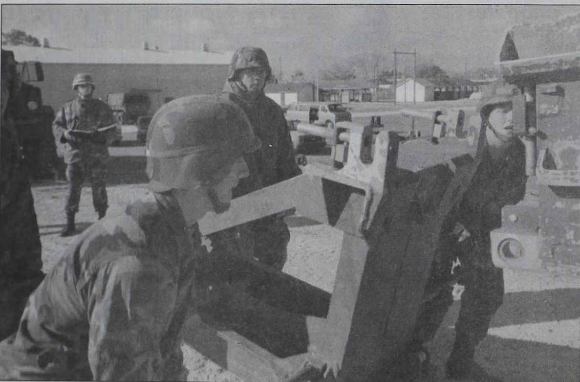
It takes four soldiers to lift the bridge's bottom panels, which weigh approximately 450 pounds each.
